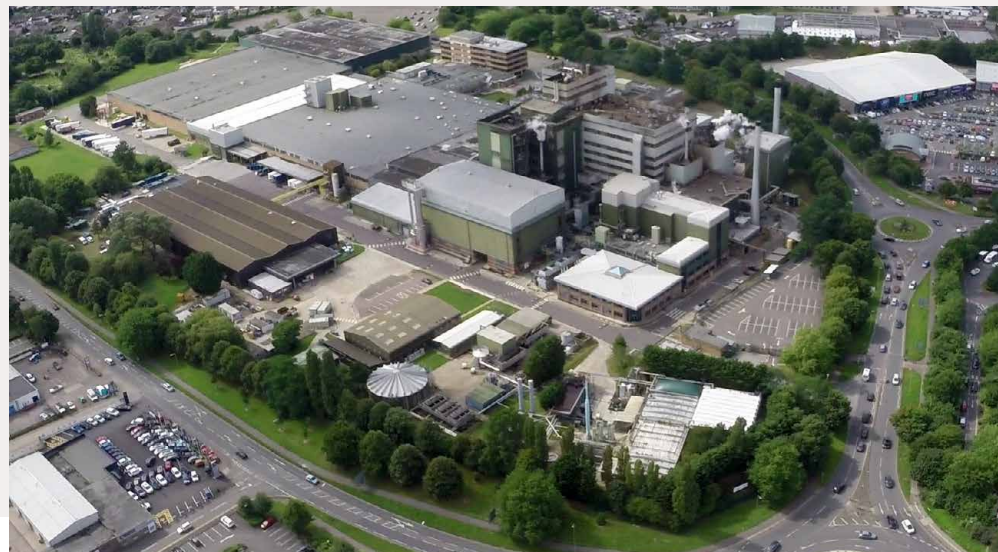
JDE manufacturing facility in Banbury, UK
